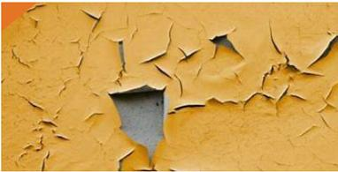
*Peeling or blistering is the lifting of the paint from the surface. This can also appear to be paint bubbles, which is fluid between dried paint.*
