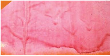
*Sags, runs, and curtains are commonly found on vertical or curved surfaces when the downward movement of paint and coatings pool immediately after application. If the paint or coating is allowed to dry with these defects they result in cracking and peeling.*
